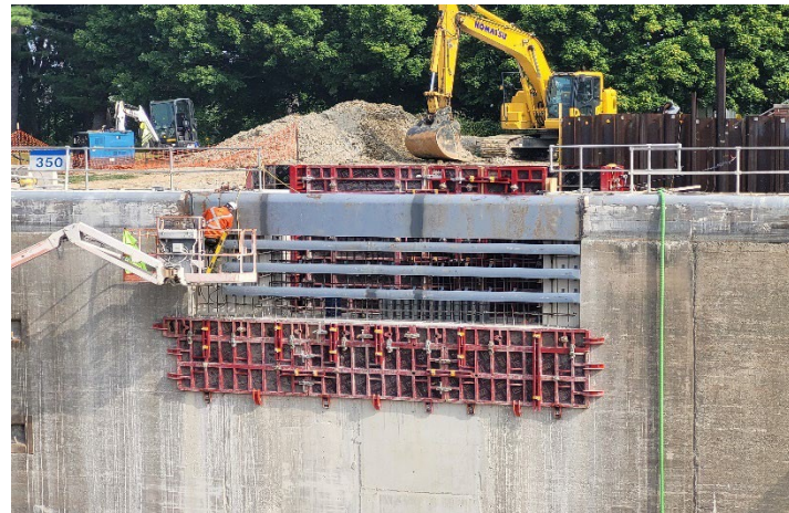
Marseilles Crossover Formwork
