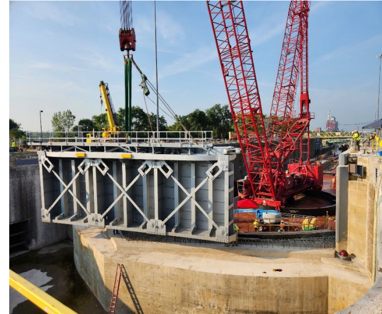
Brandon Road Miter Gate
