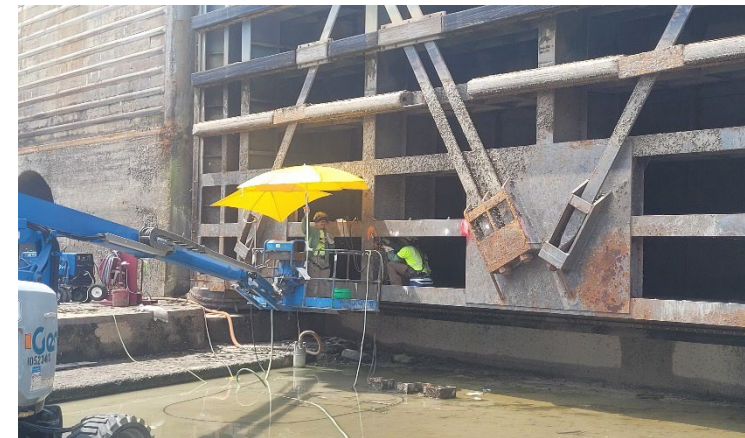
Brandon Road Miter Gate Welding
