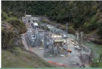
⚡ New Colgate Powerhouse
