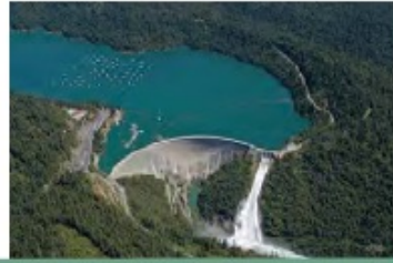
▲ New Bullards Bar Dam
