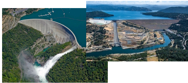
New Bullards Bar Dam Yuba River, Yuba Water Agency Oroville Dam Feather River, CA Dept. of Water Resources Sacramento District, USACE
