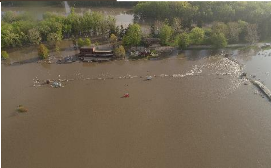
Starved Rock Lock & Dam
