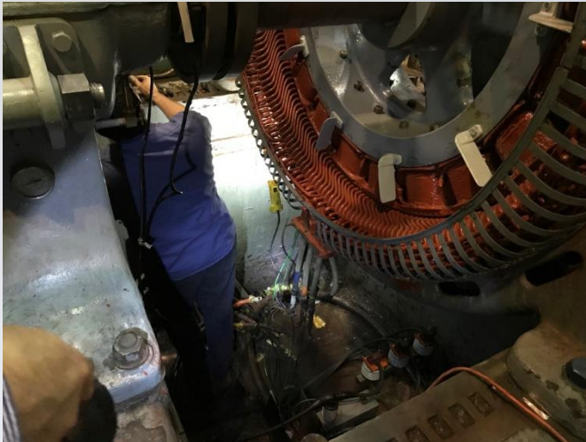
Pump and Motor Repairs
