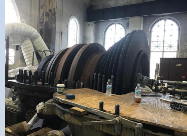
Turbine Generator 5 Repairs
