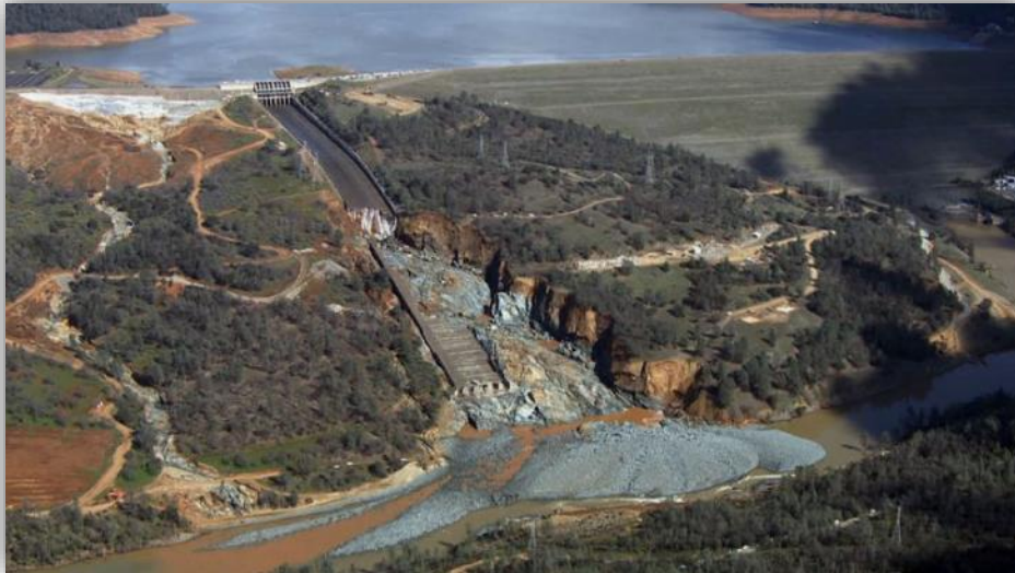
Oroville Dam, CA
