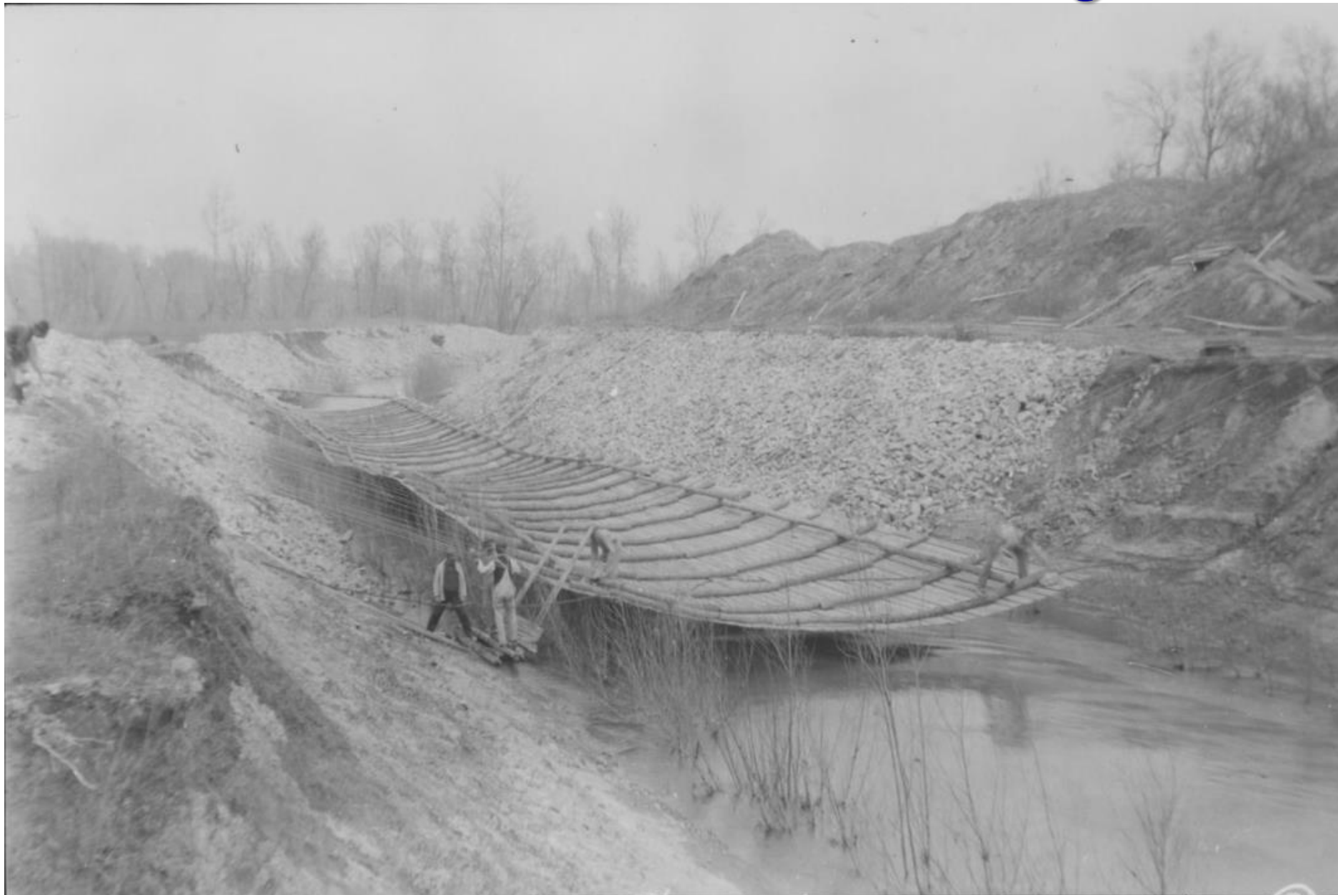
Board Mattress Sta. 640 CR. Div. Ch. Placing stone at up stream end. (2)
