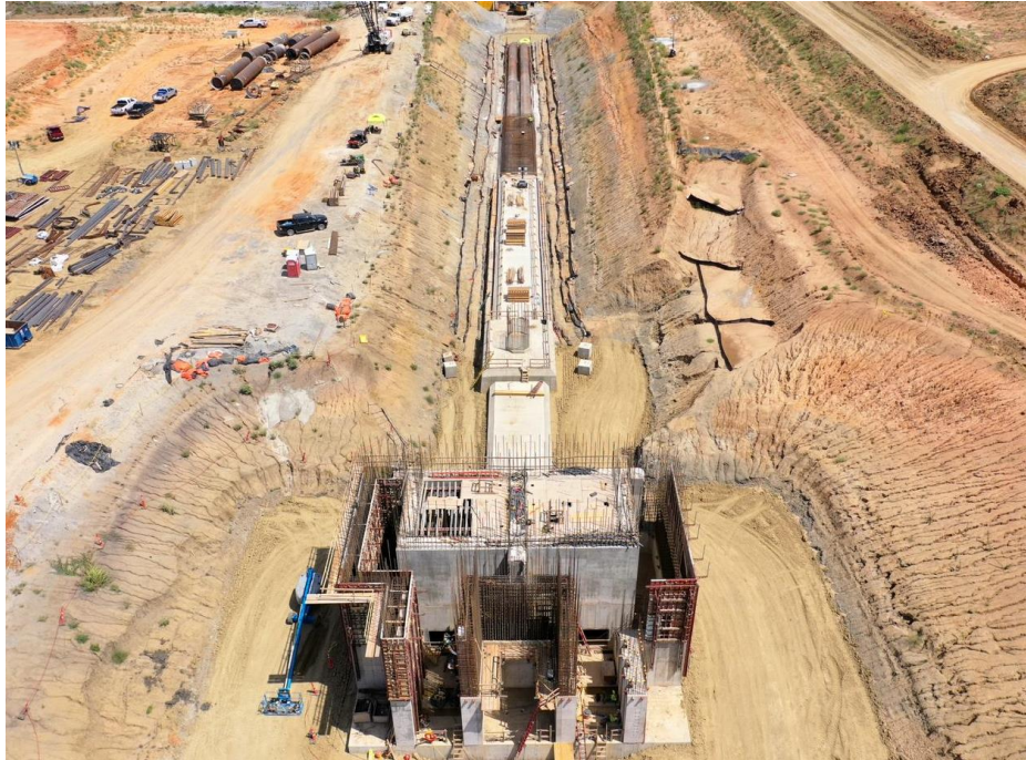
Raw Water Intake Tower – Approx. 110-feet tall when complete
