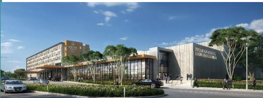
Watters Creek Convention Center – Allen
