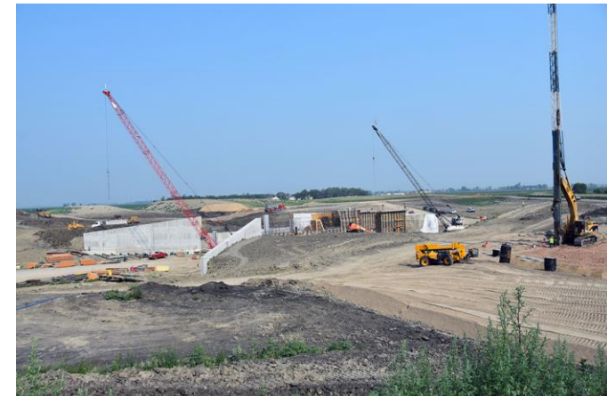
Fargo-Moorhead P3 Construction
